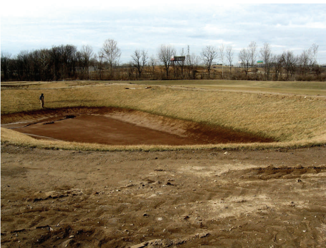
Surface Sand Filter Clogged with Construction Site Sediment, Berkeley, MO
