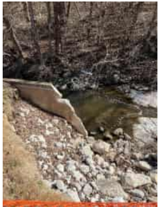
PHOTO 5.5 CREEK BANK COLLAPSE AT 1210 DES PERES AVE
