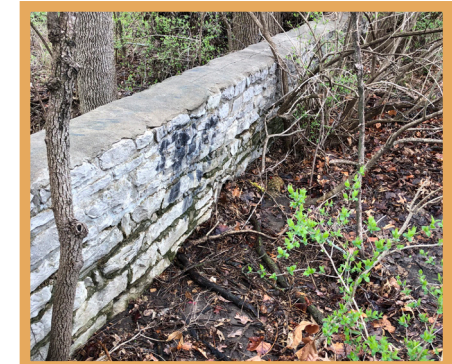
Existing Stone Wall and Drainageway
