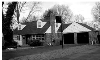
Recessed Front Entry Garage
