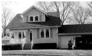
Flush Front Entry Garage
